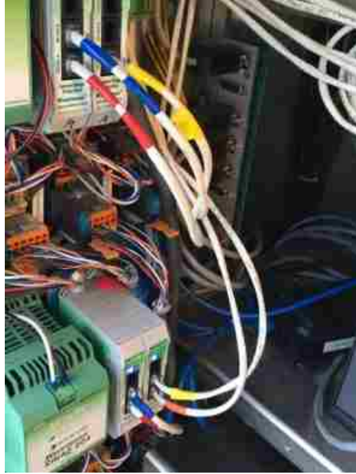
Figure 3-20: Double taped Advance cables with bridge ports above the cables (photo taken by Greg Sanchez).
