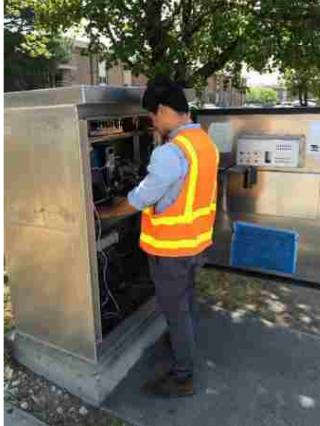
Figure 3-22: Data collector connecting the computer to the sensor (photo taken by Greg Sanchez).
